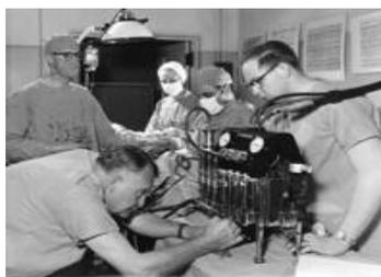
He used a blood pump he developed together with General Motors. The pump cylinders were activated by air pressure and vacuum. Dr. Dodrill did 13 procedures with this pump between July 1952 and December 1954.
